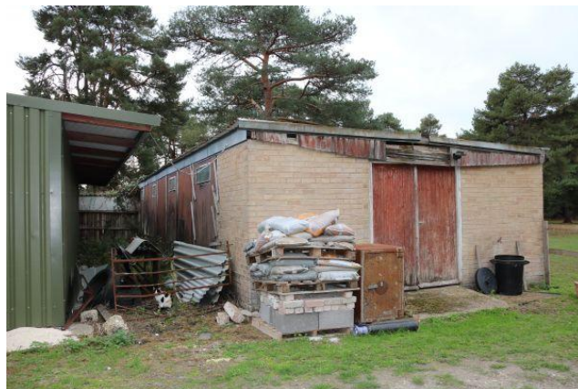
(Potential Unit 5 for renovation)
